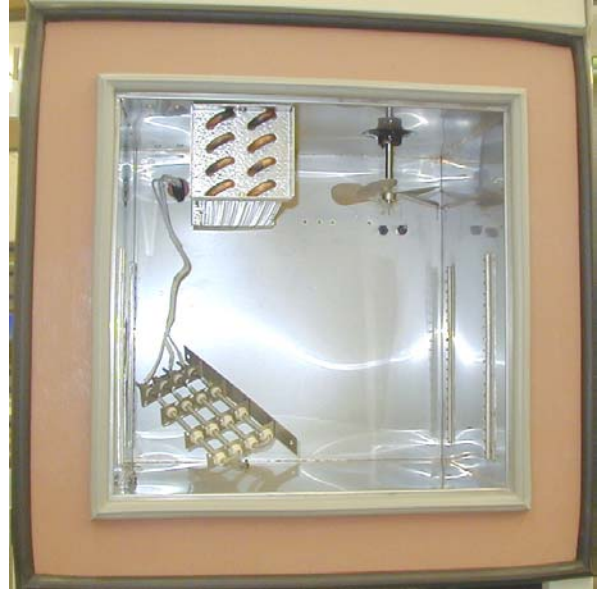
Heater Rack Removal #2
